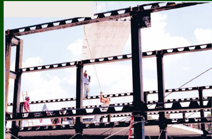
Erection of Steel Structure
