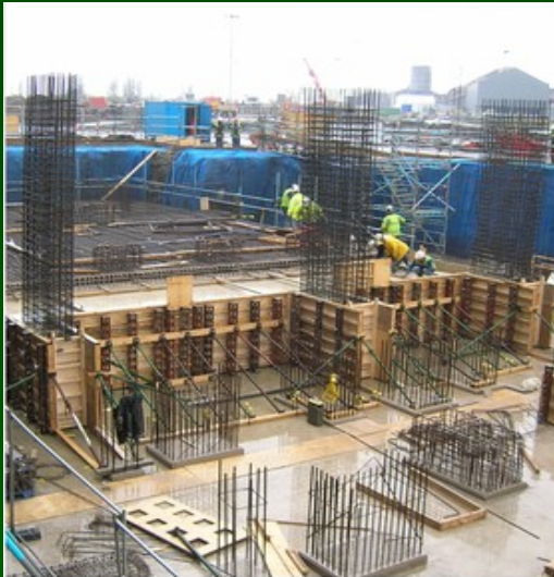
Erection of Concrete Structure
